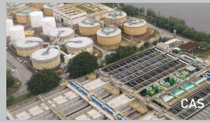
Sewage treatment area
